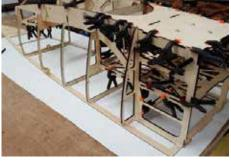
Once all Glued. Add F7 & F8 to fuselage 3MM Shape ( Super Glue is fine for this)
